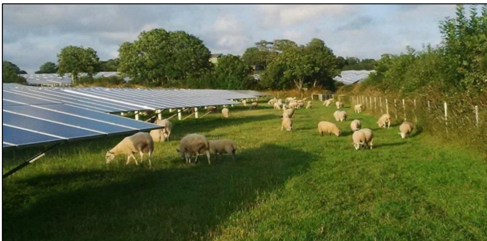
Figure 8.4: Ground Coverage Under Arrays - Example
