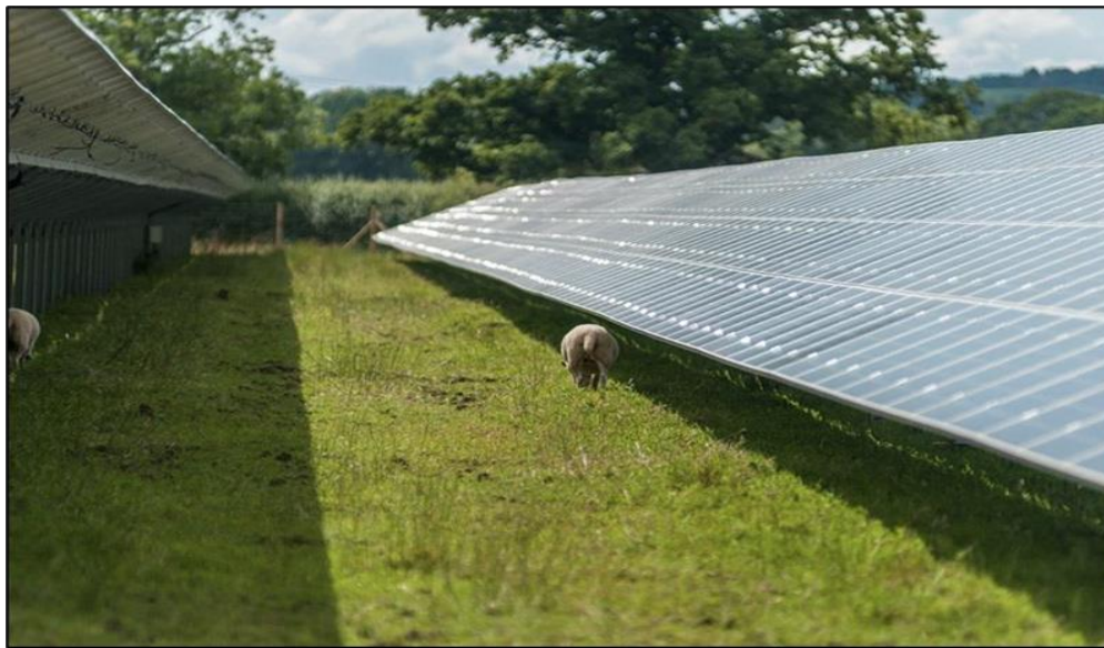
Figure 8.5: Ground Coverage Under Arrays – Example 2
